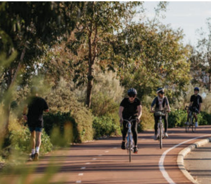
Bi-directional coated asphalt shared path. The red coating is more fitting with a heritage aesthetic than traditional uncoated asphalt - riverfront bike path, Perth WA
