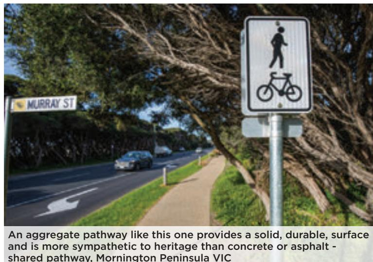
An aggregate pathway like this one provides a solid, durable, surface and is more sympathetic to heritage than concrete or asphalt - shared pathway, Mornington Peninsula VIC
